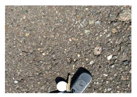
Figure 3: Example of Loss of mastic, raveling (3yr, WI 190/94)
